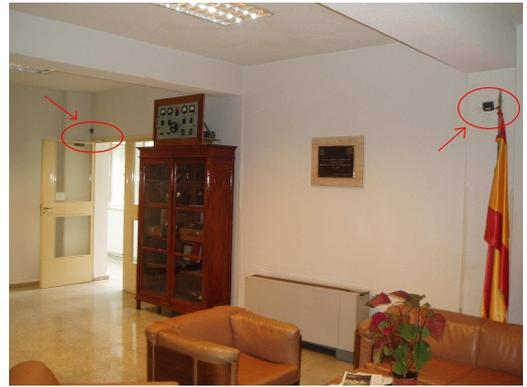
Fig. 1. PLACEMENT OF THE RFID TAGS ON THE WALLS AT A HEIGHT OF 2 M.
